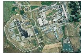
A bird's eye view of the Washington State Reformatory
